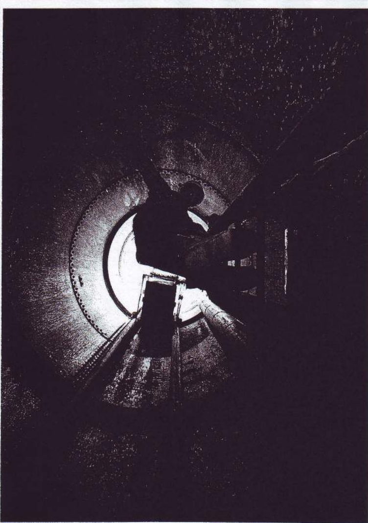
Interior of Borehole 10X is lined with old railroad tank cars eight feet in diameter and made of thick steel.
